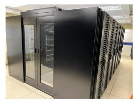
Inside the HEPIC-IFUSP Building on the first floor is hosted CCIFUSP data center, which is designed to separate the cold corridor from the hot corridor
