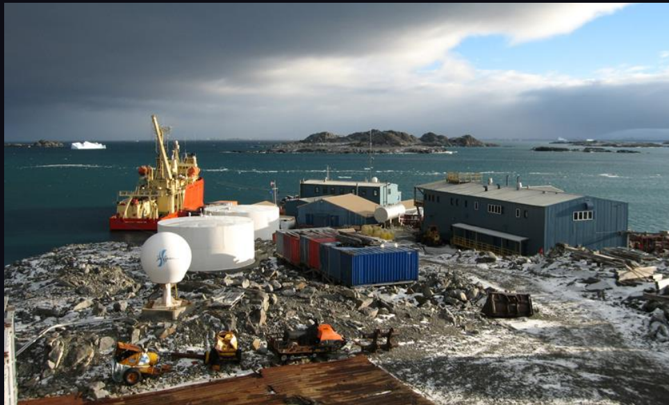
Radionuclide station RN73, Palmer Station, USA, CTBTO
