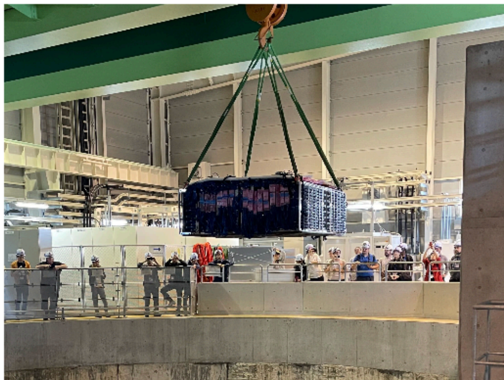
(iv) Installing the detector into the pit by a crane
