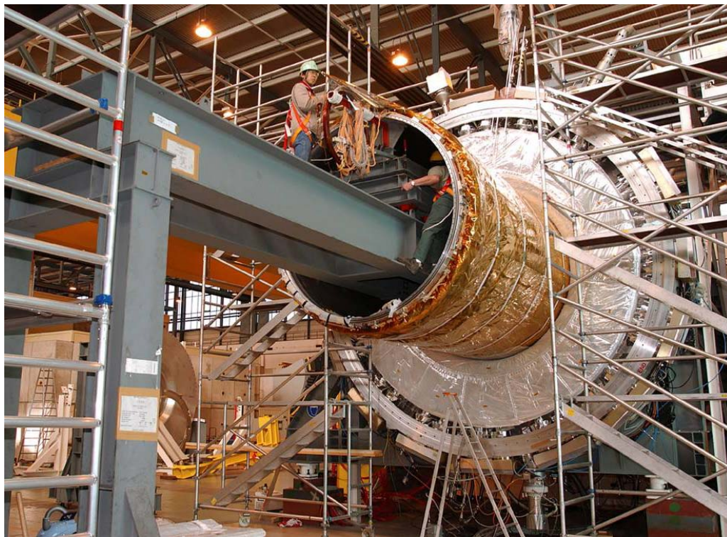
Solenoid insertion into the barrel LAr vessel
