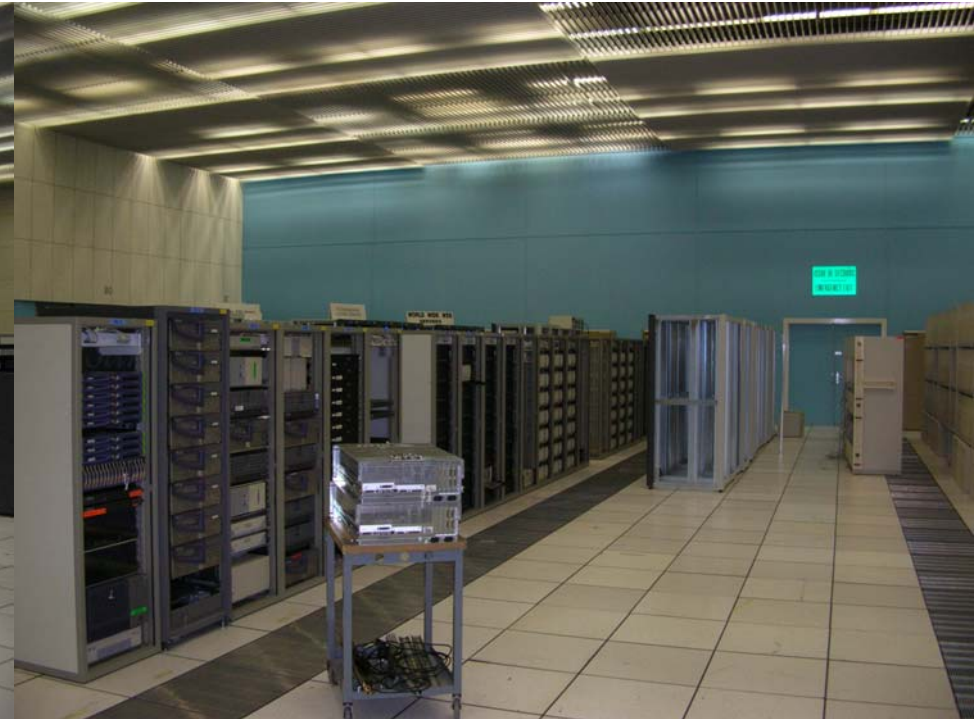
New structure on the already refurbished right side
