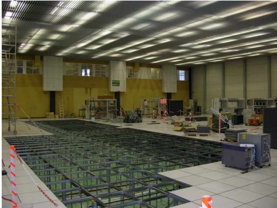
Refurbishment of the left side of the Computer Center has started
