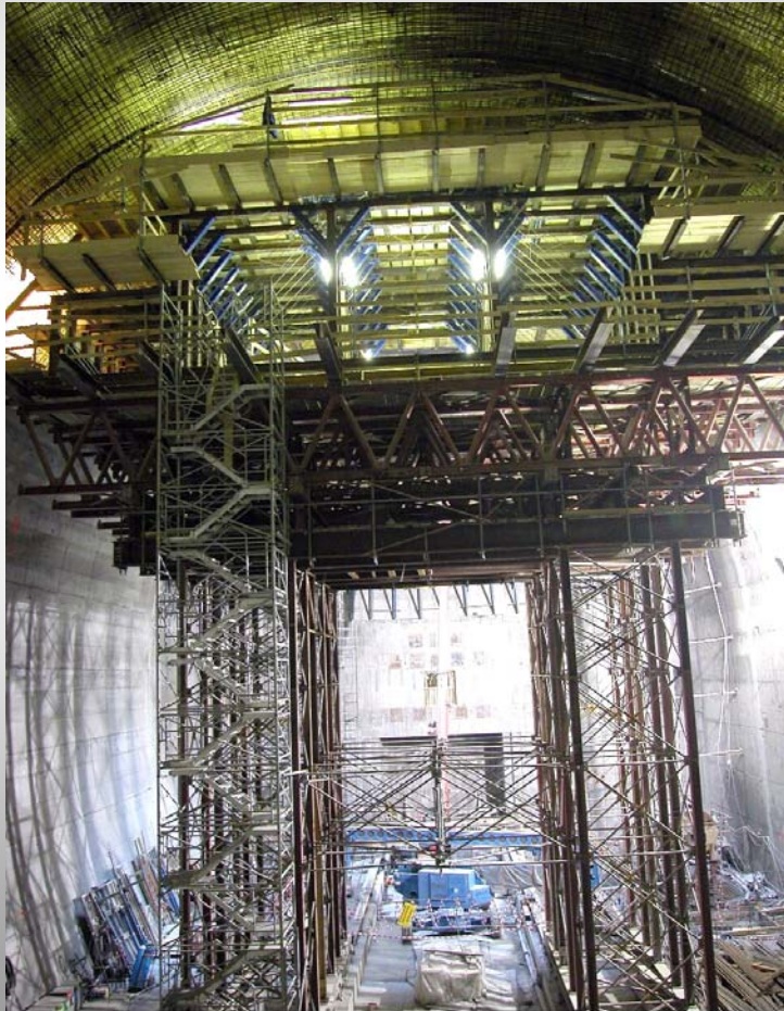
LHC Point 5 - UXC55 Cavern - Crown Reinforcement fixing - 23-02-2004 - CERN TS/CE
