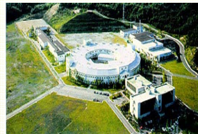
Large-scale Research Equipment (Pohang Synchrotron Lightsource Accelerator)
