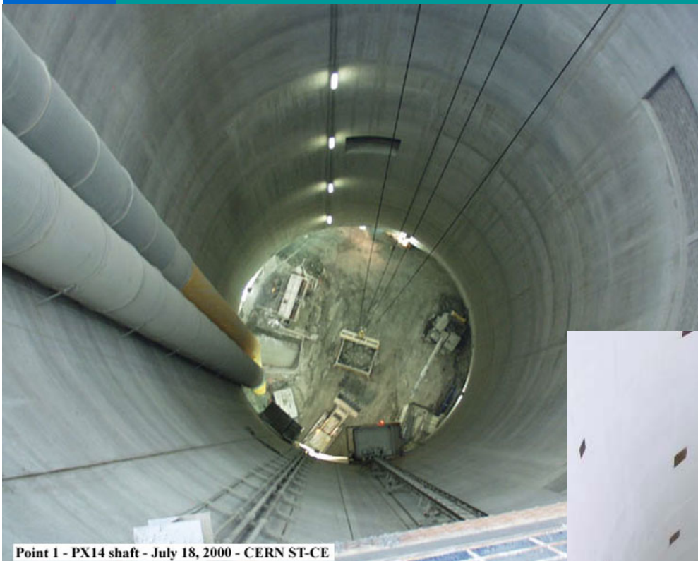
Point 1 - PX14 shaft - July 18, 2000 - CERN ST-CE
